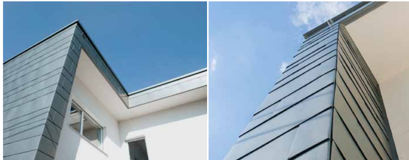
Grey Skin Natural House. Standort Padova, PD Planer Arch. Matteo Rampin Baujahr 2017
